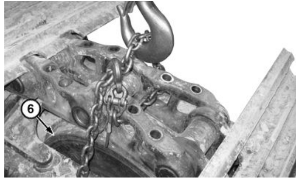
Track Chain Removal
