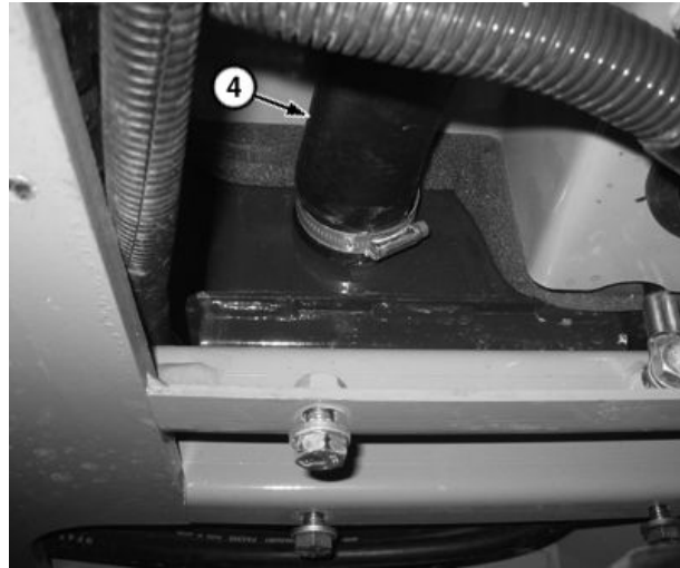
Hydraulic Oil Supply Line
